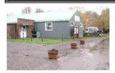
THE CAR PARK to the village hall was regularly run over by passing vehicles with the result that large puddles formed. Road planings have been rolled into the puddles and half barrels put on top.
